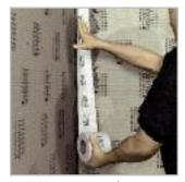
$\begin{array}{ll} \mbox{DRY-DB(V)} - \mbox{integrating sealing tape into} \\ \mbox{wall} / \mbox{floor connections} \end{array}$
