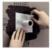
DRY-DBWM — sealing pipe duct
