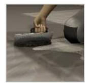
$\label{eq:decomposition} \mbox{DRY-ASK} - \mbox{filling wall and floor surfaces}$
