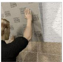
ELEMENT-EL — for application on walls (e.g. as wall levelling over existing tile coverings) ...
