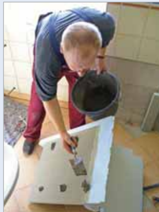
■ Dots of LUX ELEMENTS®-COL-AK fixing adhesive are applied on the rear of the cladding where the holes have been drilled.
