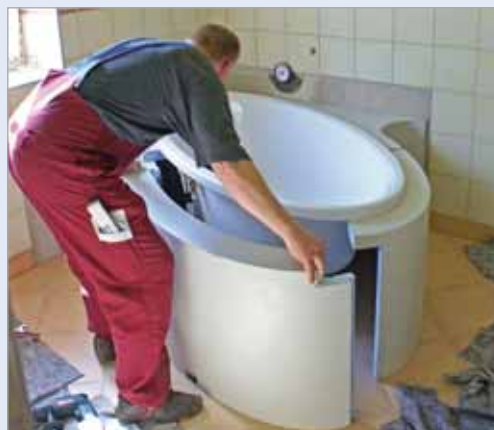
■ The bath tub is inserted when all fixed parts are anchored. The pipes are connected afterwards and the remaining loose elements are glued to the elements anchored on the wall. The right adhesive LUX ELEMENTS®-COL-PU is used for this.
