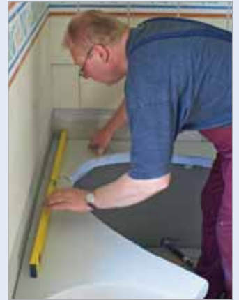
■ Step by step installation: The craftsman level the prefabricated parts with a spirit level. He checks the dimensional and fitting accuracy.
